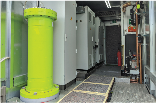
Stornetic high-speed flywheel: Internal view of the plant with the flywheel (green), power converter (on the left), and cooling system (on the right)
