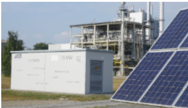
Compact Lithium-Ion-Storage in KITs research environment
